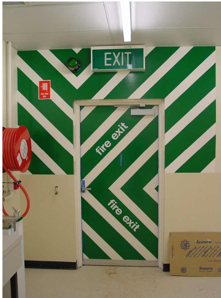
Photo 1: DHUD exit identification
